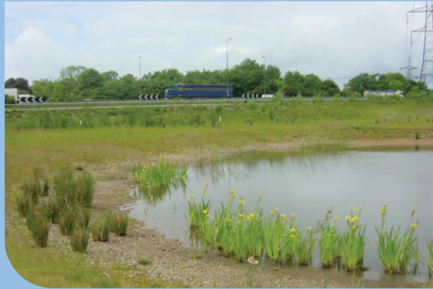
A balancing pond - one of the methods used to treat water run off from roads
