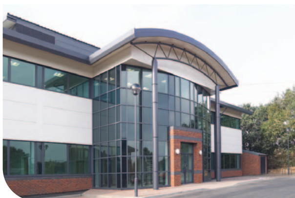
National Traffic Control Centre at Quinton, near Birmingham
