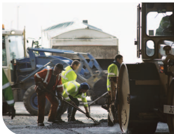
Highways Agency contractors at work
