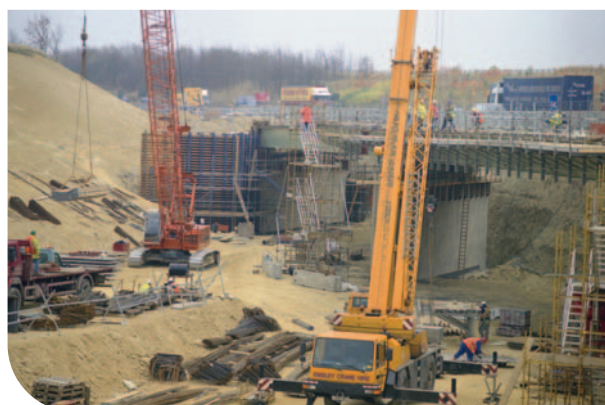
Example of contractor's at work on the Agency's network
