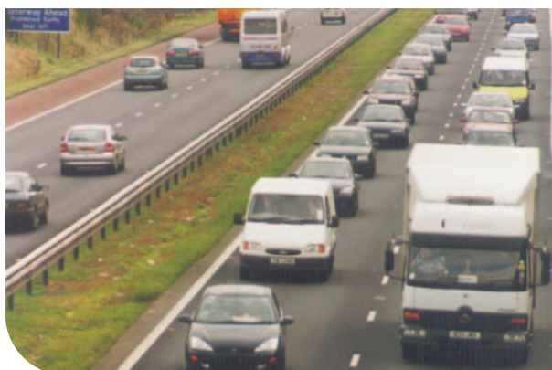
Congestion on the A74 North of Carlisle
